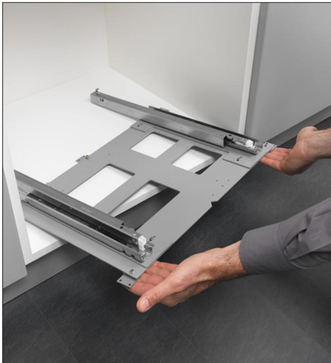
Position the runner support at the centre of the cabinet, using the front reference. The front feet, aligned with the base panel of the cabinet, can be used as a reference for the depth positioning.
